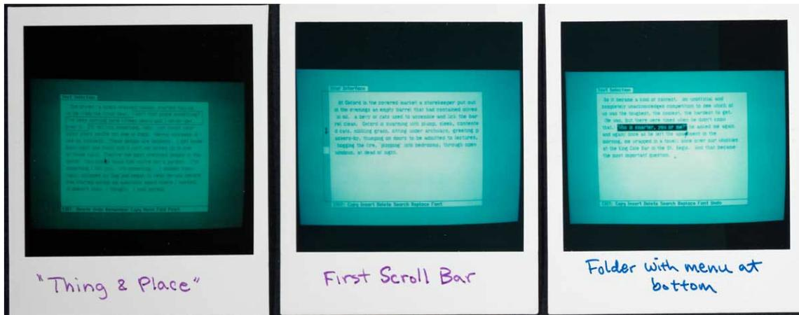
By now, it's the spring of 1980 and things are starting to happen fast. The leftmost picture shows the earliest text selection, using a different highlighting technique than we ended up with. It also shows a "command bar" at the bottom of the screen, and that we had started to use non-modal commands (make a selection, then perform an action, instead of the other way around).
